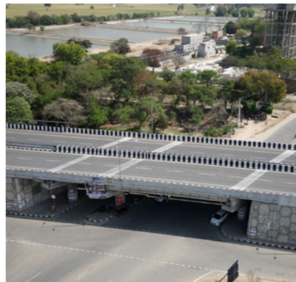
Construction of 6-lane Greenfield Varanasi-Ranchi-Kolkata Highway (Package 11)
