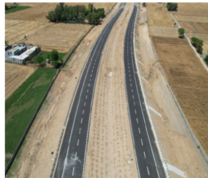
Construction of four-lane Greenfield Delhi-Amritsar-Katra Expressway (Package-II)
