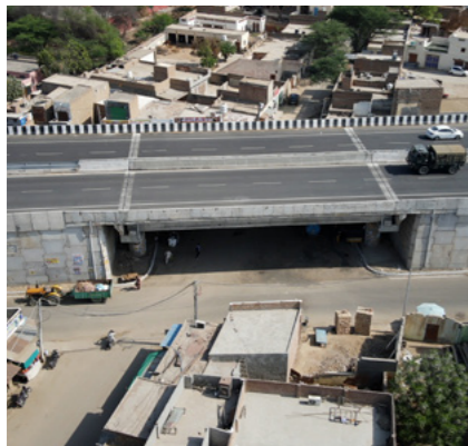
Construction of 6-lane Greenfield Varanasi-Ranchi-Kolkata Highway (Package 12)
