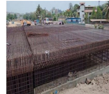
Design And Construction of 4 Nos. Structures on Gonde-Vadape Section of NH-3
