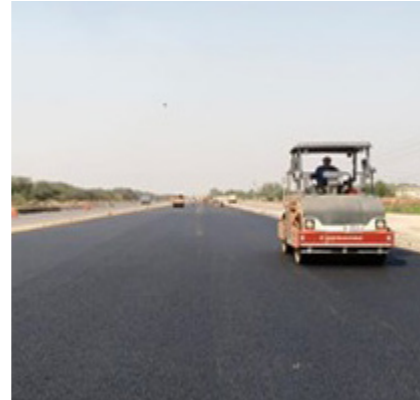
Development of 6-lane access controlled Ludhiana-Bathinda Greenfield highway section of NH-754AD
