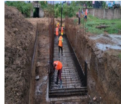
Construction of Four Lane Elevated Corridor in Danapur-Bihta Section, Bihar
