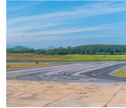
Resurfacing of Runway and Aircraft Operating Area at AF Station Halwara
